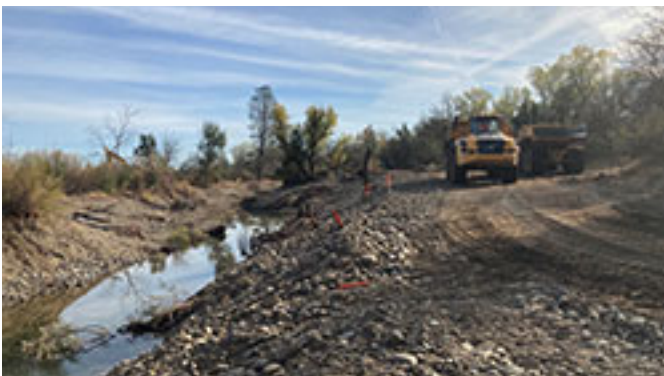
Creating three meandering side channels off the Sacramento River near Anderson has involved heavy construction and earth-moving equipment over the past 12 months.
